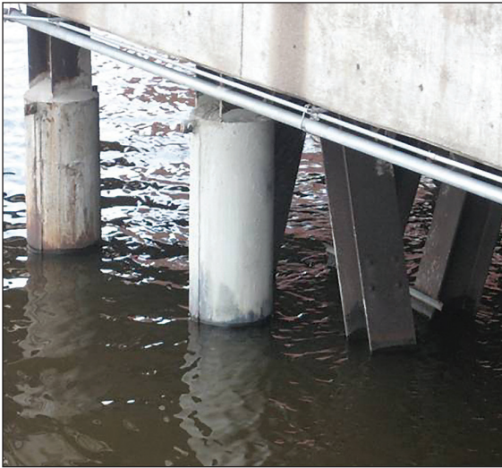
Figure 13: Steel jacket option shown on steel pile (Gene Clark/UW Sea Grant Institute).
