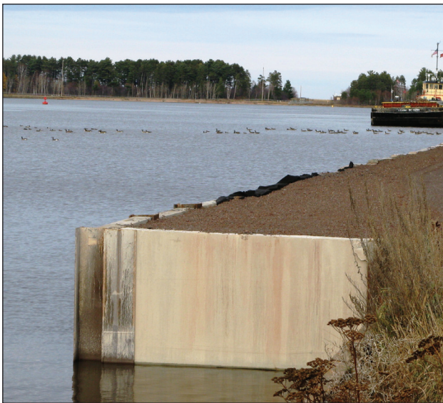
Figure 12: A new wall in front of a failed timber structure (Chad Scott-AMI Consulting Engineers).
