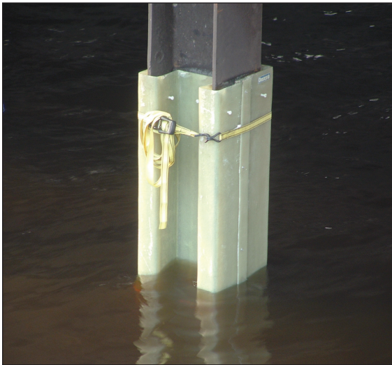
Figure 14: Fiberglass jacket option shown on steel H-pile (Gene Clark/UW Sea Grant Institute).
